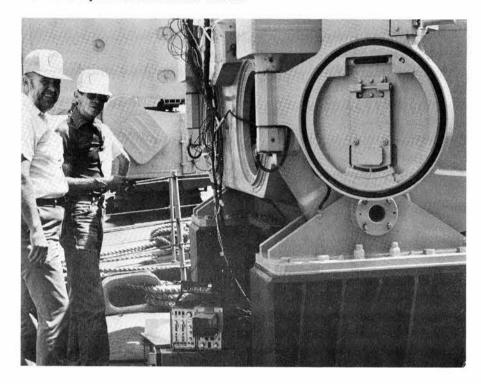
ROSS YINGST and Jim Gearhart, right (both 5132), are installing connecting cables between armored box launcher for cruise missiles and Sandia test equipment on the deck of the destroyer *U.S.S. Merrill.*
